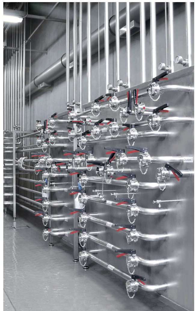
ASI-BUS-ES control head KI-TOP with selective emergency cut-off and 2 freely assignable control inputs
