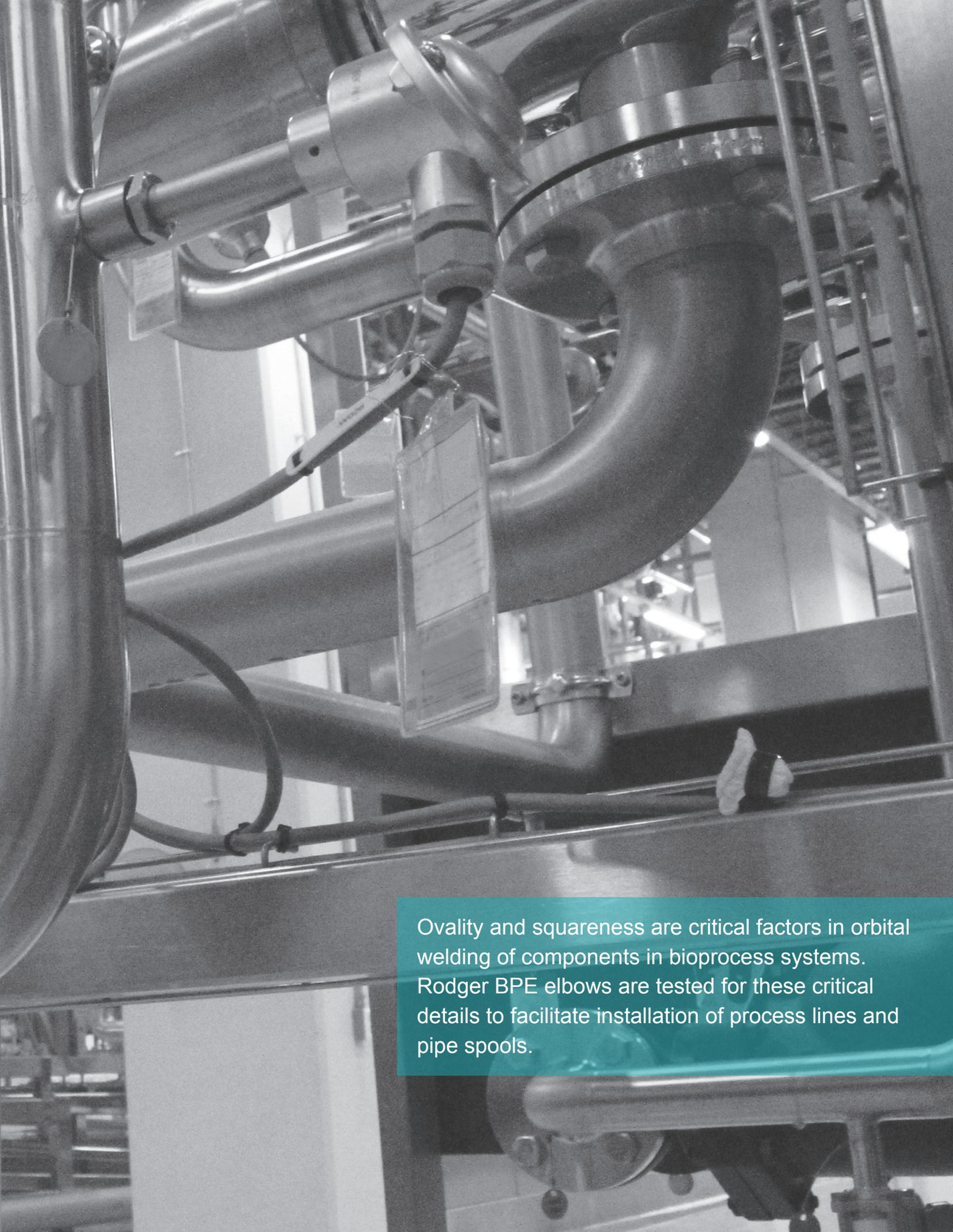
Ovality and squareness are critical factors in orbital welding of components in bioprocess systems. Rodger BPE elbows are tested for these critical details to facilitate installation of process lines and pipe spools.
